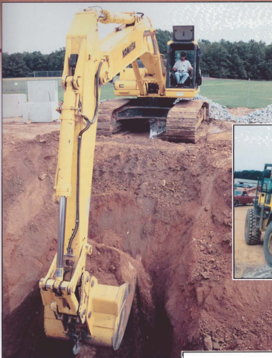
Crews from Mount Construction used a large fleet of Komatsu equipment on a recent expansion project at Edgewood High School in Berlin, New Jersey. This included (clockwise from above left), the operator of a Komatsu PC400LC-6 excavator cutting a deep utility trench; the operator of a WA250 wheel loader stockpiling aggregate; and the operator of a D61 dozer using the machine's blade for grading.
