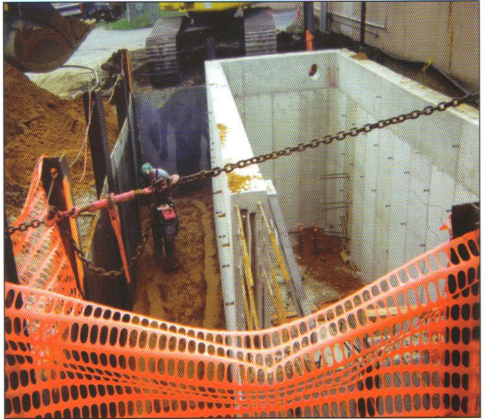
Installation of concrete sludge tank in Mt. Holly.
